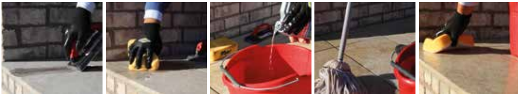
PIC 1. Fill joint with grout.
