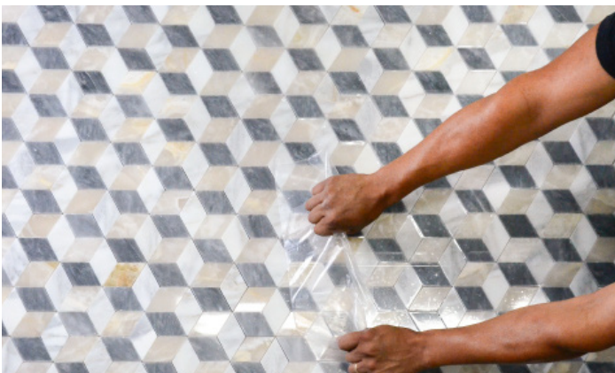
Step 5 After 24 hours of cure time, peel the tape from the tile, starting from the corner. Use an angled, downward movement.
