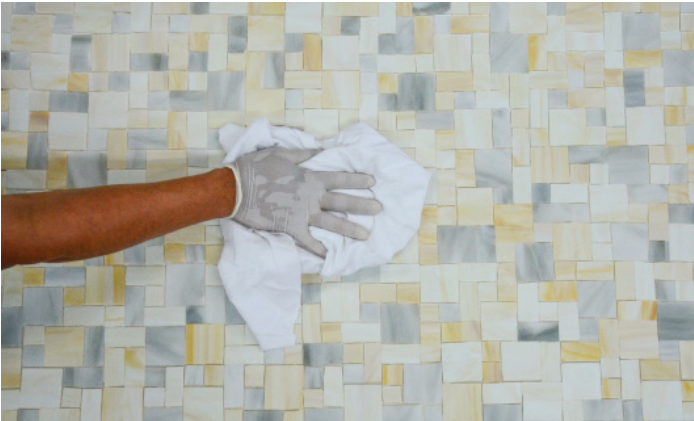
Step 8 Remove excess sealer with a clean white cloth. Allow cure time per manufacturer's instructions.
