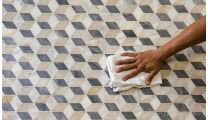
Step 10 For final removal of grout haze, polish with a clean, soft, white cloth.
