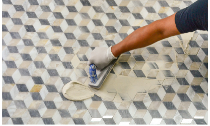
Step 8 Apply grout with a rubber grout float, forcing grout into joints until full. Remove excess grout with edge of float.
