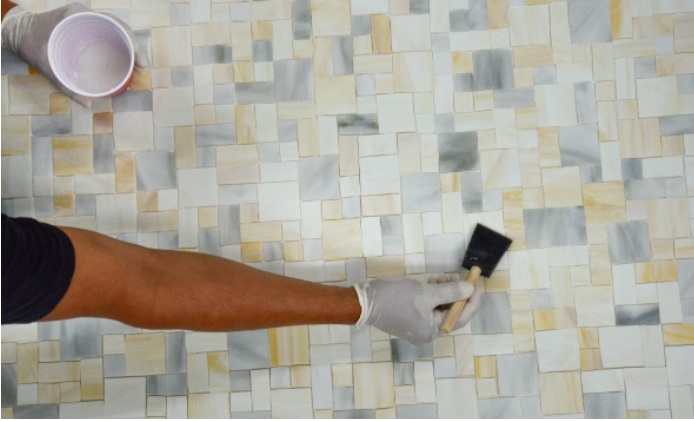
Step 7 Apply Oceancare penetrating sealer as grout releases, per manufacturer's instructions.
