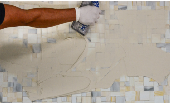
Step 9 Apply grout with a rubber grout float, forcing grout into joints until full. Remove excess grout with edge of float.
