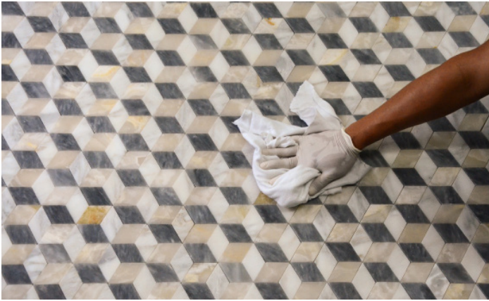
Step 7 Remove excess with a clean white cloth. Allow cure time per manufacturer's instructions.
