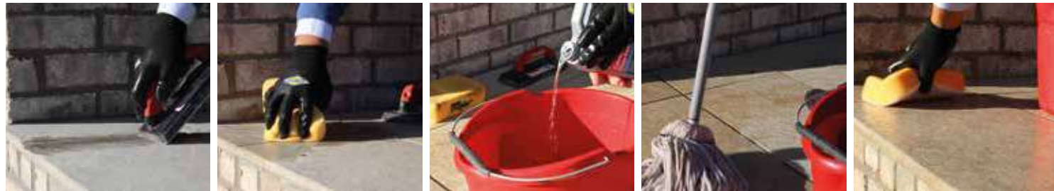
PIC 1. Fill joint with grout.
